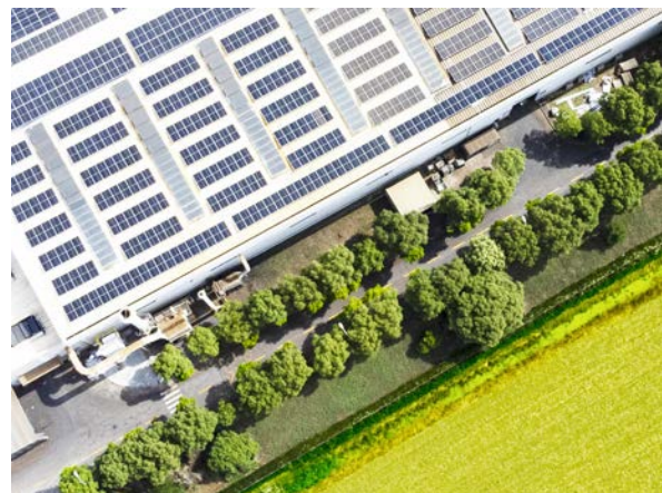
GF Casting Solutions installed 2.0 MW of roof-mounted PV capacity, such as this 1.4 MW system on the iron foundry in Kunshan (China).
